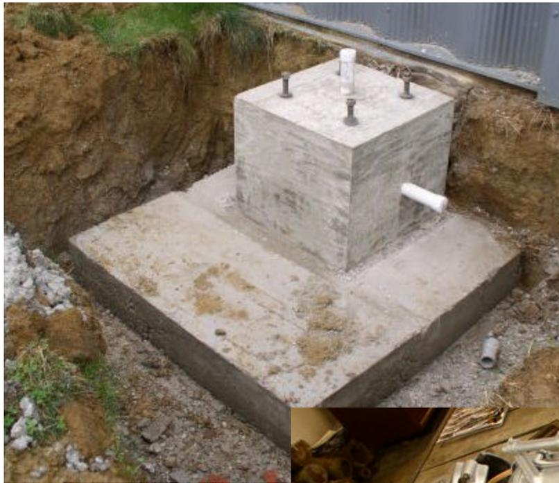
Starting at the bottom was the need for a very solid base on which to secure the upright signal post.
